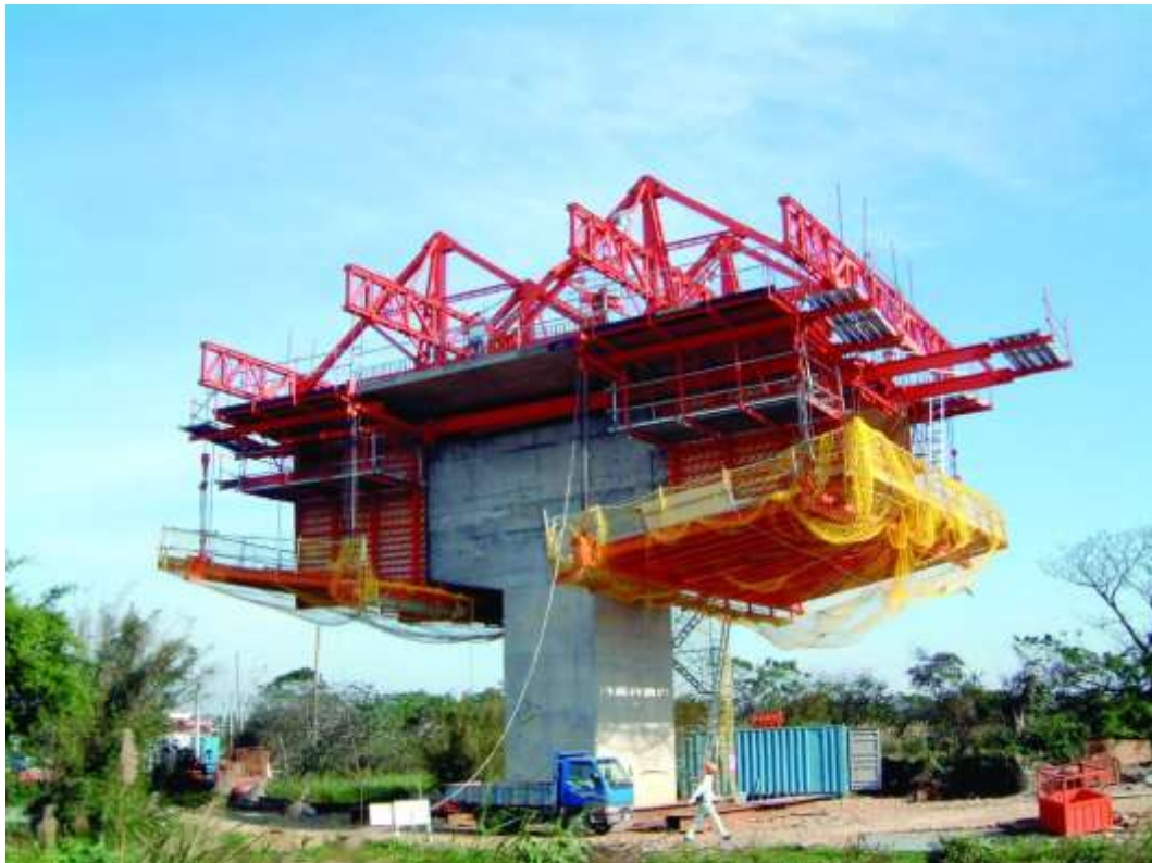
Figure 2.10: Travelling Formwork
